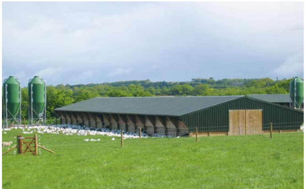
Green silos, green sheds and green trees can all help get the go-ahead for new projects.
